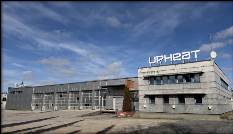
Upheat factory in Tampere, Finland
